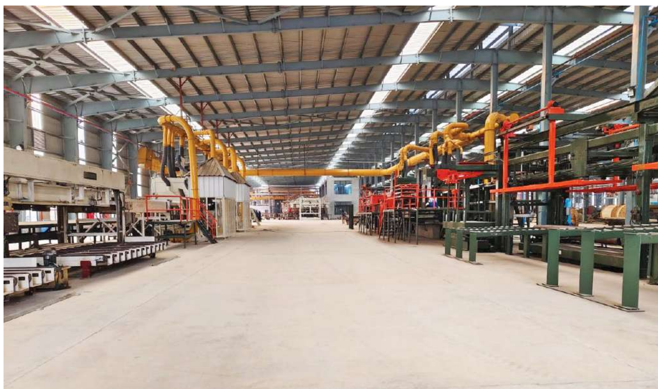
Fervent Multiboard Industries Limited - Multi Board manufacturing plant at Jamalpur Economic Zone (Under Implementation)
