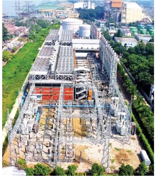
United Ashuganj Energy Limited - a 195 MW gas based IPP Power Plant at Ashuganj, Brahmanbaria
