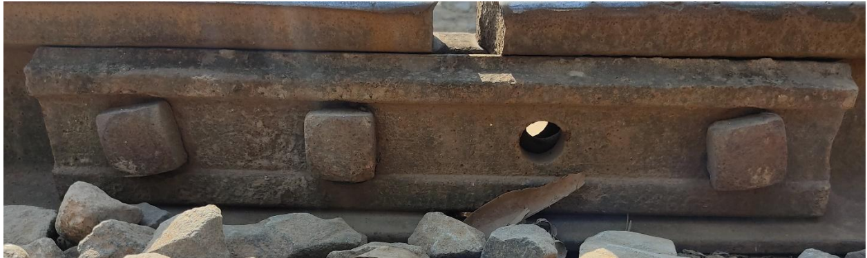
Fig.12 Defective Fishplate
