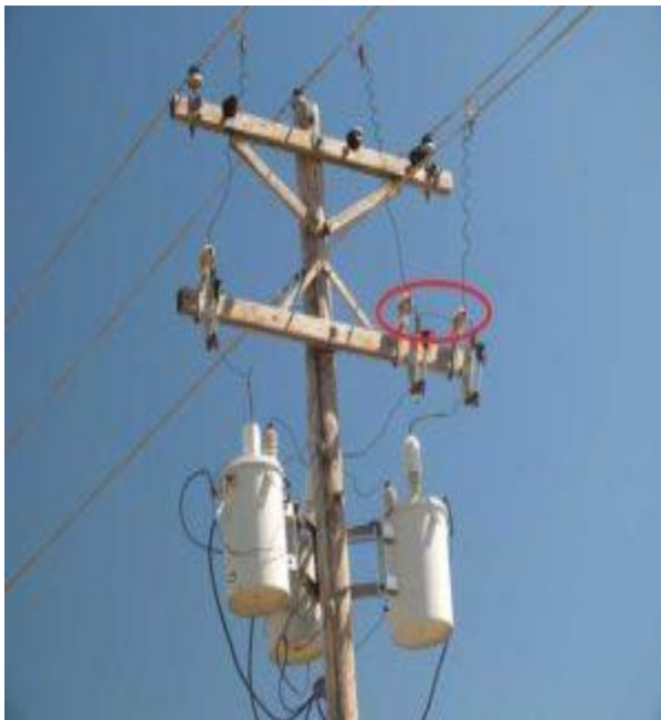
Fig 3.2: Lightning arrester
