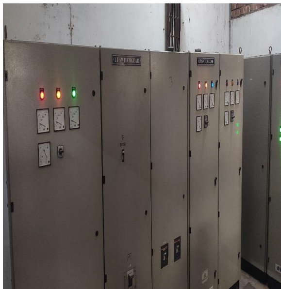
Fig 2.2: LT switch gear
