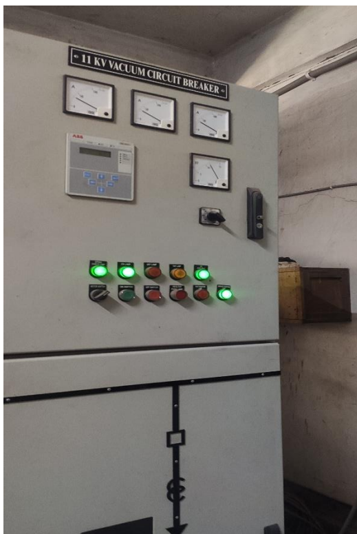
Fig 2.3: Vacuum circuit breaker
