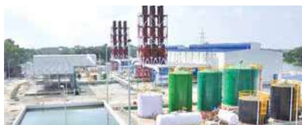
Orion Power Meghnaghat Ltd. financed by Agrani Bank PLC.
